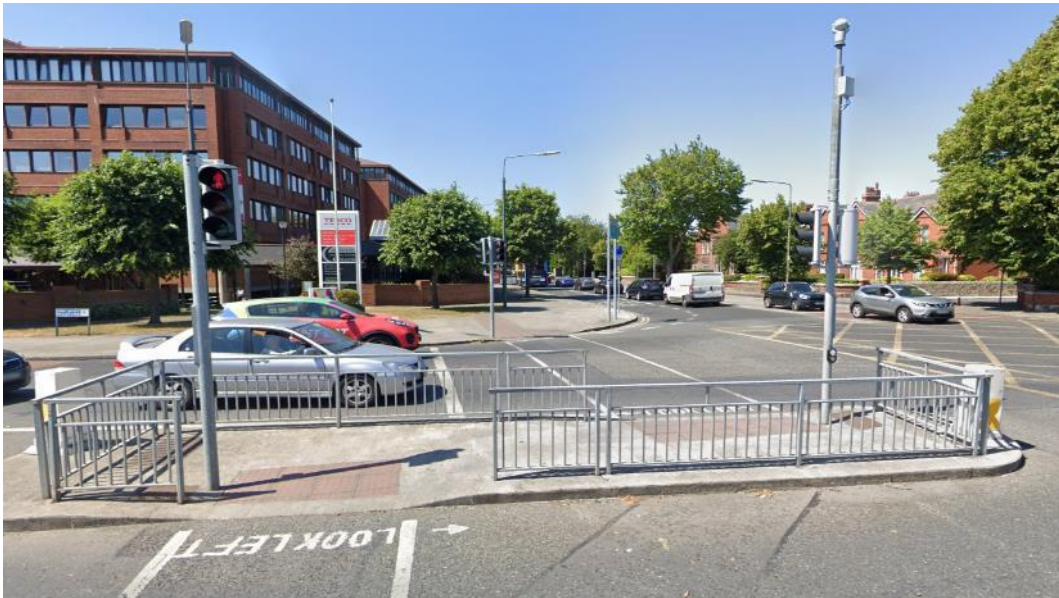
Figure 90: Tactile Paving Surface at Pedestrian Island – Nutley Lane
