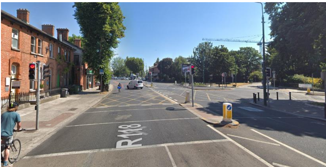
Figure 32: Pedestrian Crossing Point with Pedestrian Island – Ballsbridge
