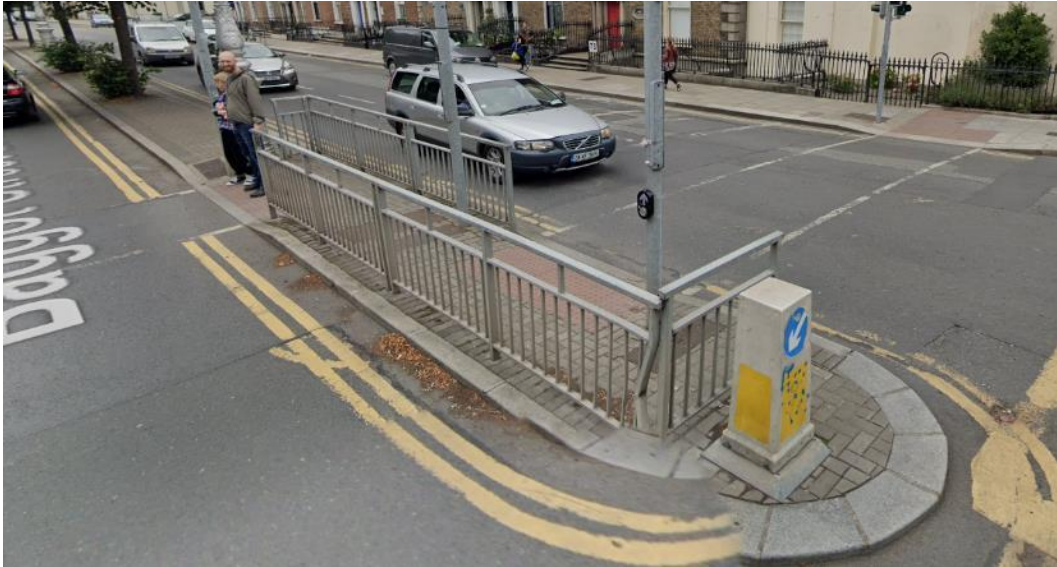
Figure 67: Tactile Paving Surface at Pedestrian Island – Baggot Street Lower
