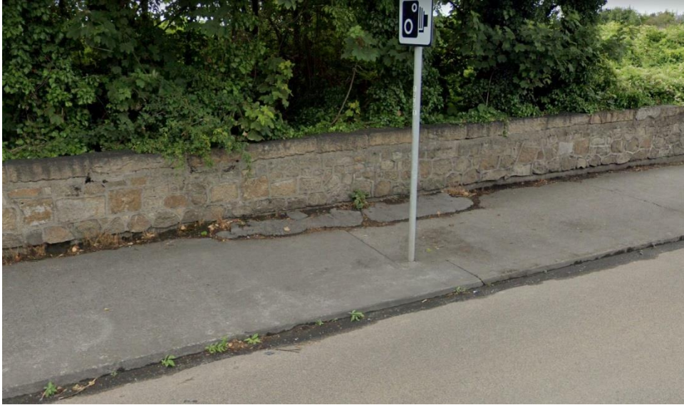
Figure 16: Example of poor-quality patch repair - Merrion Road
