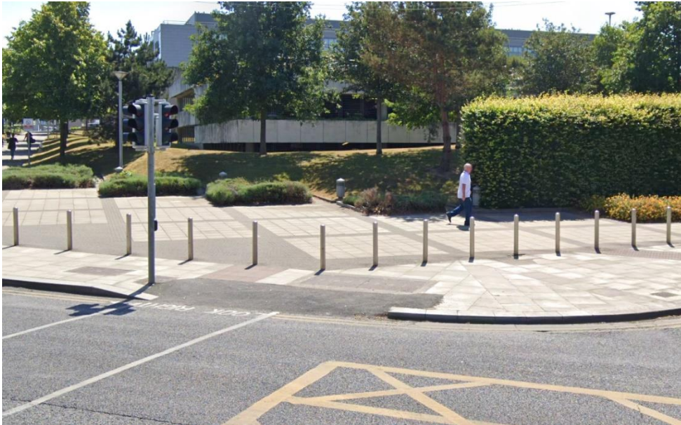
Figure 20: Controlled Crossing - Merrion Road, Nutley Lane junction
