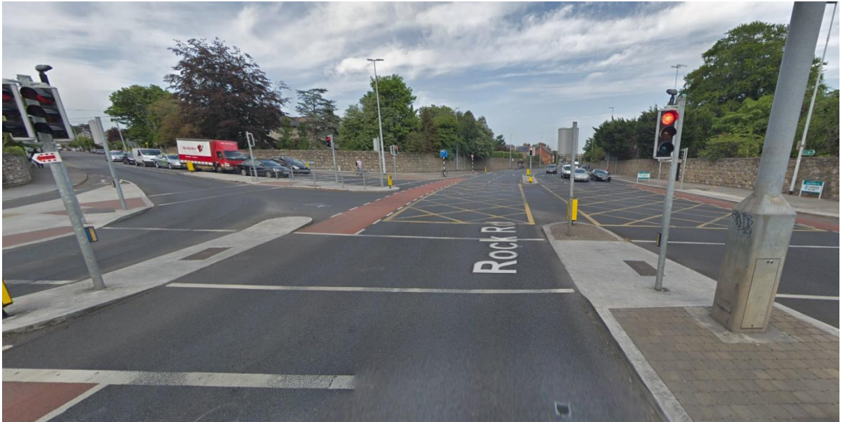
Figure 10: Tactile Paving - Rock Road
