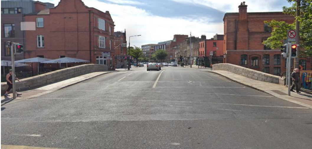
Figure 69: Level Change – MacCartney Bridge (Baggot Street Bridge)
