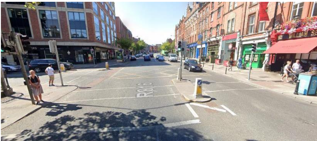
Figure 64: Pedestrian Crossing Point with Pedestrian Island – Baggot Street Upper
