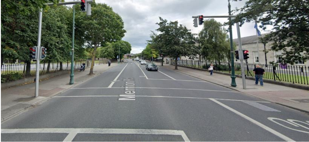
Figure 39: Tactile Paving Surface – Merrion Road
