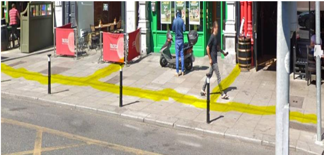
Figure 57: Drainage Channels – Baggot Street Upper
