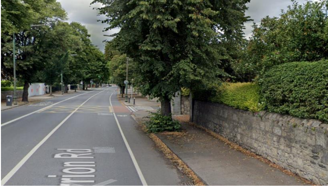
Figure 50: Tree reducing footpath effective width – Merrion Road
