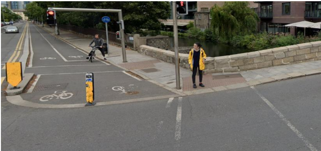
Figure 70: Shared Surface – MacCarthy Bridge (Baggot Street Bridge)
