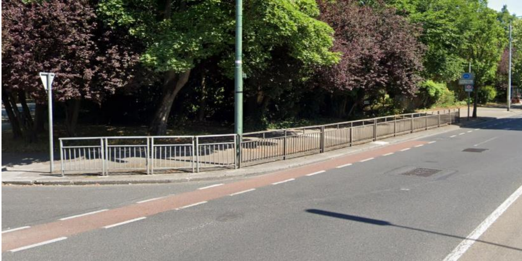
Figure 31: Guardrails – Merrion Road
