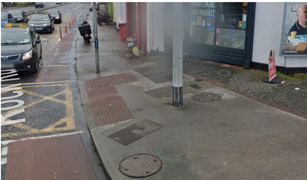
Figure 11: Tactile Paving - Rock Road / Booterstown Avenue
