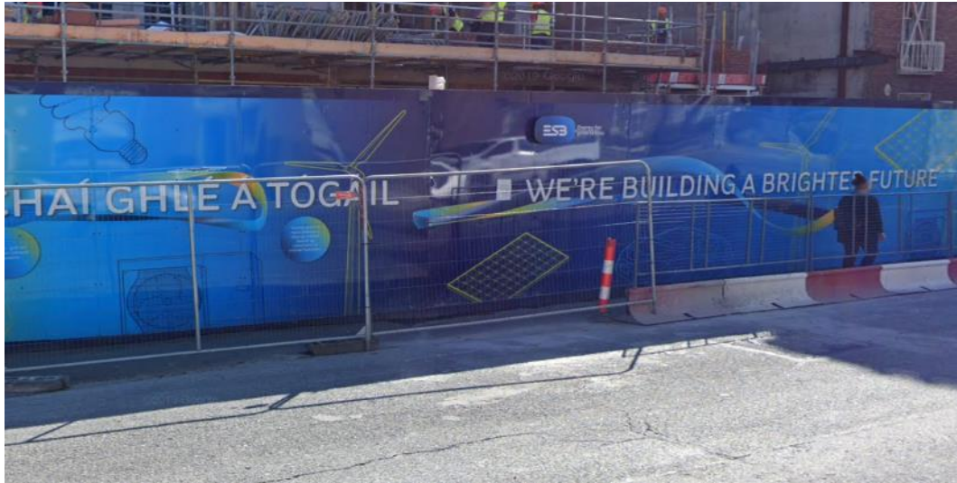
Figure 60: Temporary Guardrails – Fitzwilliam Street Lower
