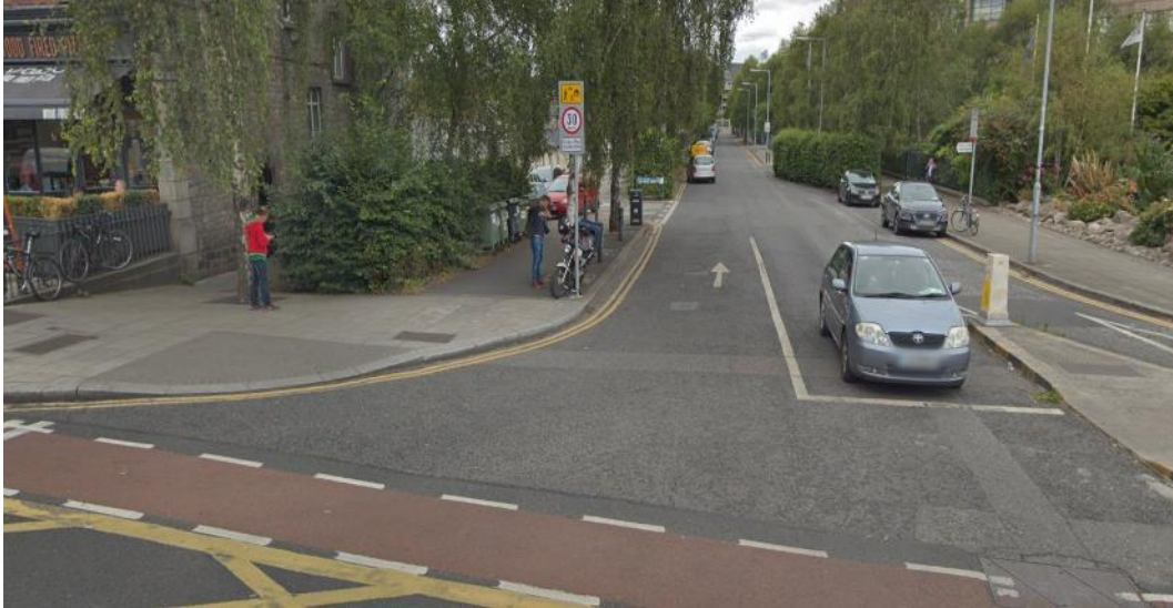
Figure 37: Uncontrolled Crossing Point with Dropped Kerb on Curve of Road – Merrion Road / Ballsbridge Park Junction
