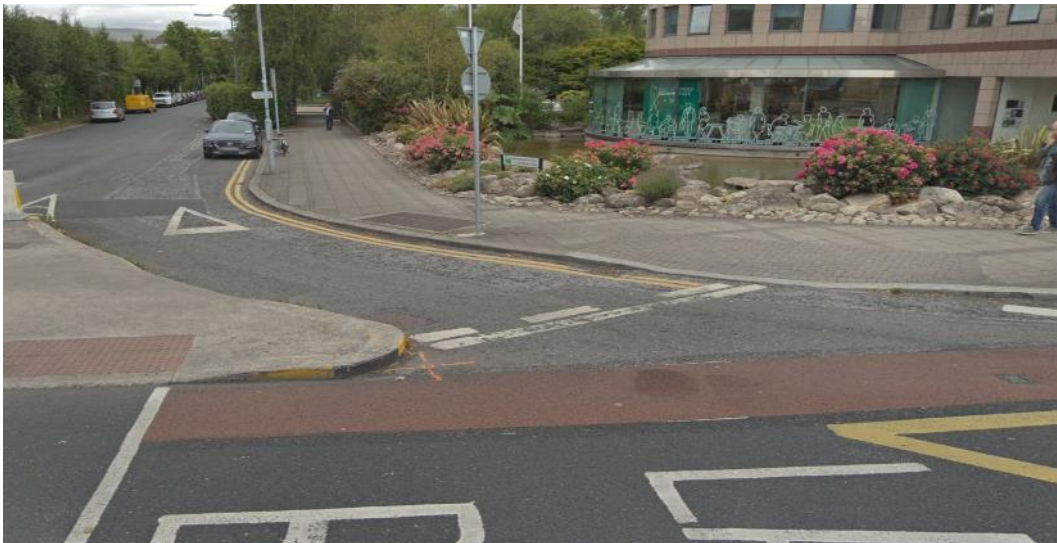
Figure 38: Uncontrolled Crossing Point with Dropped Kerb on Curve of Road – Merrion Road / Ballsbridge Park Junction
