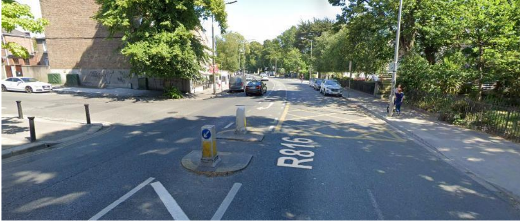
Figure 65: Pedestrian Crossing Point with Pedestrian Island – Pembroke Road
