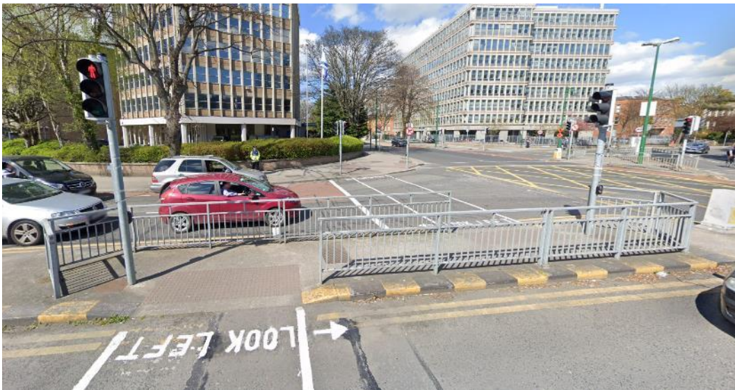
Figure 59: Guardrails – Pembroke Road
