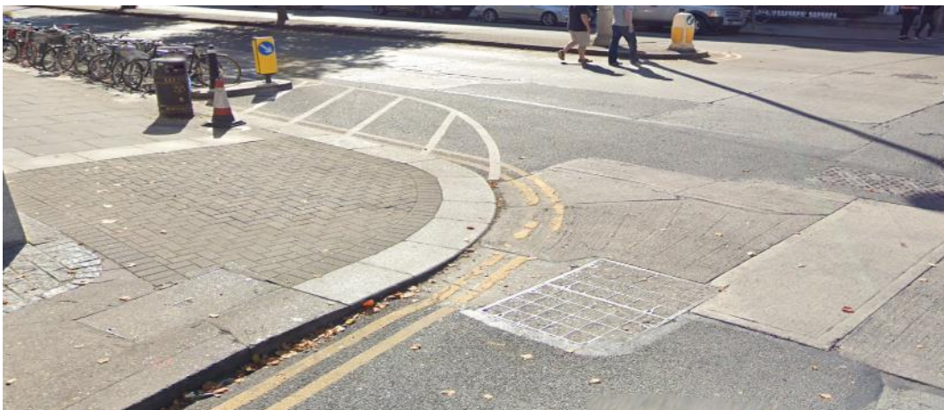
Figure 66: Uncontrolled Crossing Point with Dropped Kerb on Curve of Road – Baggot Street Lower
