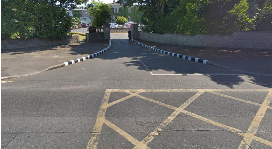
Figure 89: Uncontrolled Crossing Point with Dropped Kerbs on Curve of Road – Nutley Lane
