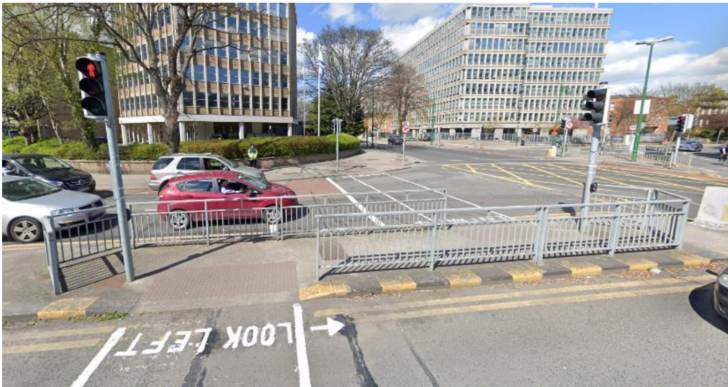
Figure 68: Tactile Paving Surface at Pedestrian Island – Pembroke Road
