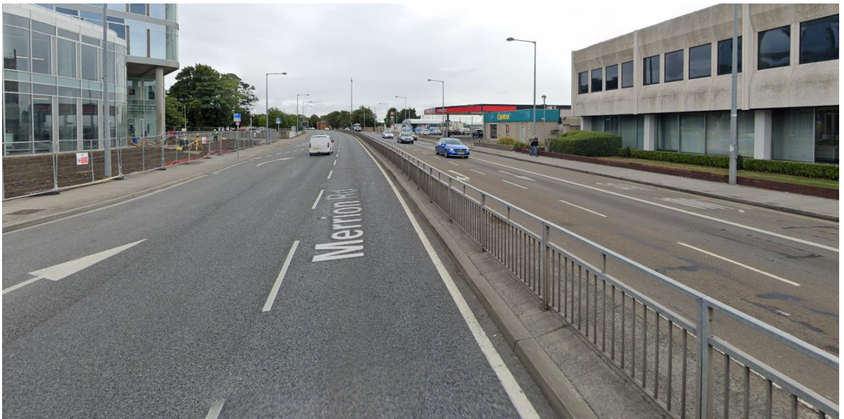
Figure 18: Guardrail - Merrion Road
