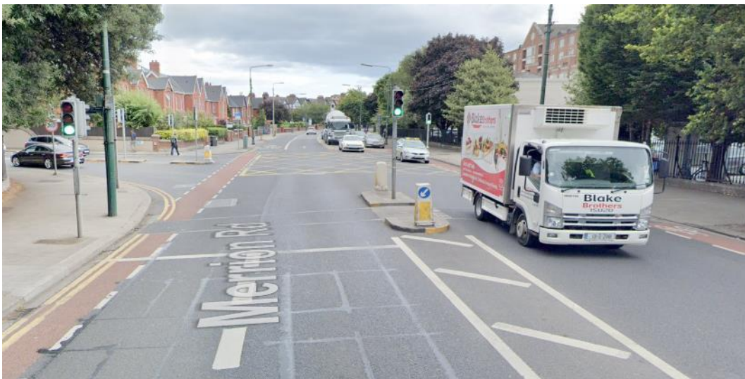
Figure 41: Controlled Junction without Tactile Paving Surface – Merrion Road
