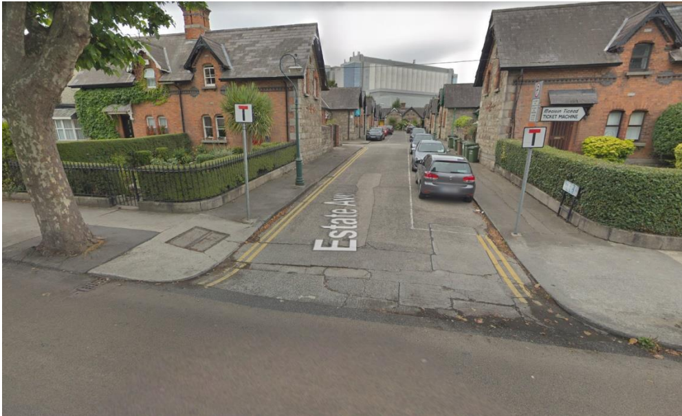
Figure 23: Surface Material - Merrion Road
