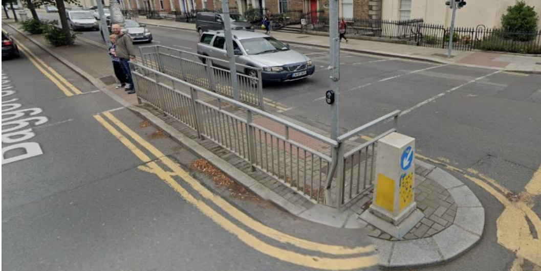
Figure 58: Guardrails – Baggot Street Lower
